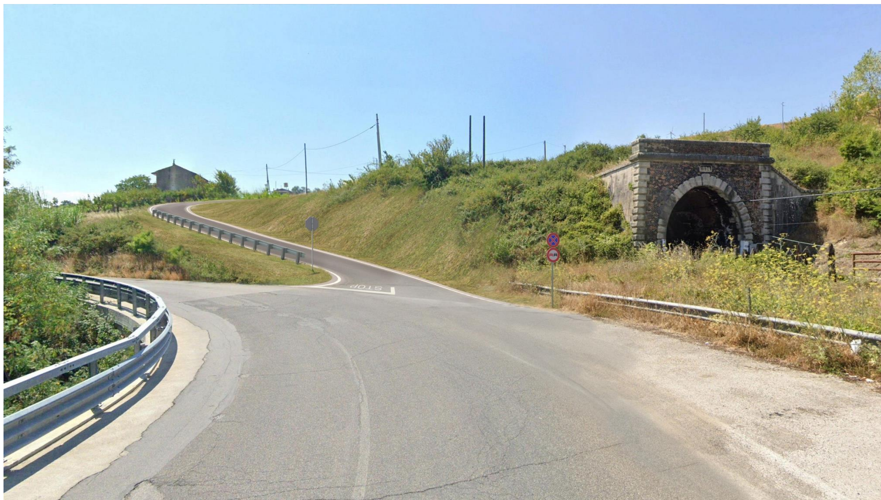
Figura 8-3 Post operam intervento NV22
