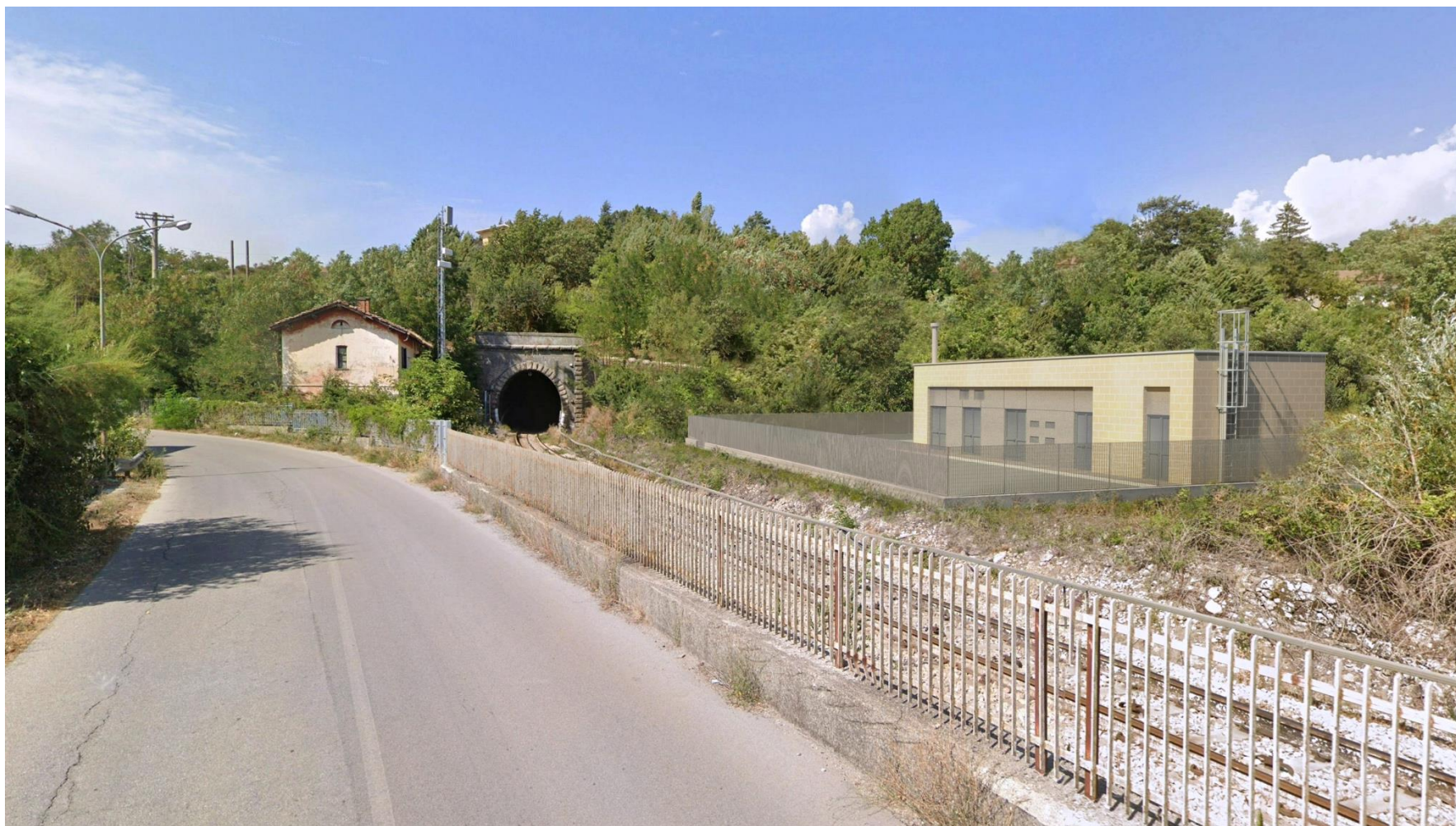
Figura 9-3 Post operam intervento NV23
