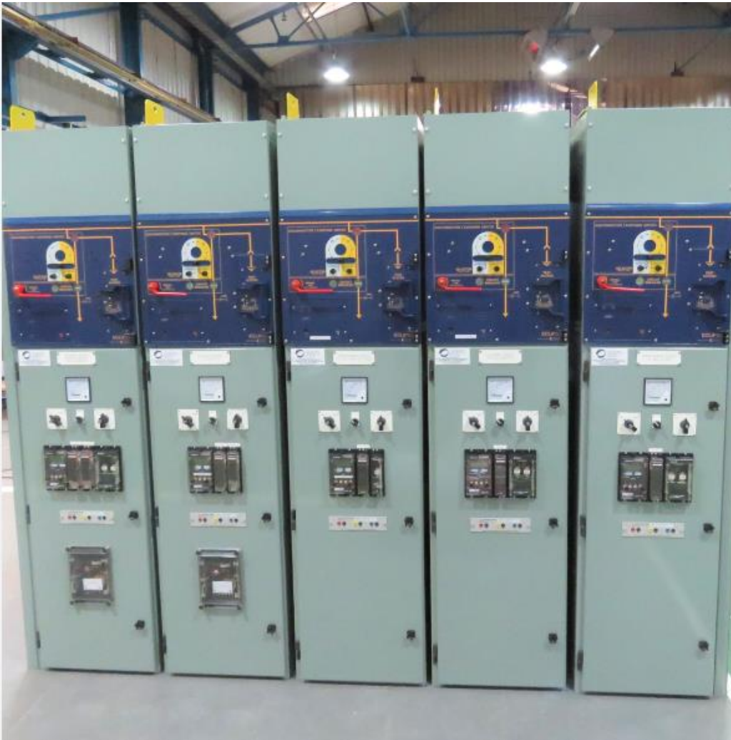
Figura 7 – MV switchgear
