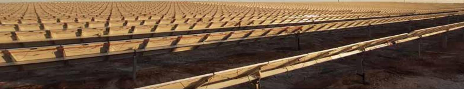
**Track** Horizontal single-axis trackers increase the performance of PV power plants by up to 30% with a limited increase of the investment. By following the sun throughout the day PV trackers maximise power generation. They also better match the grid demand profile, which peaks in the afternoon, and contribute to a smarter and more sustainable energy system.
