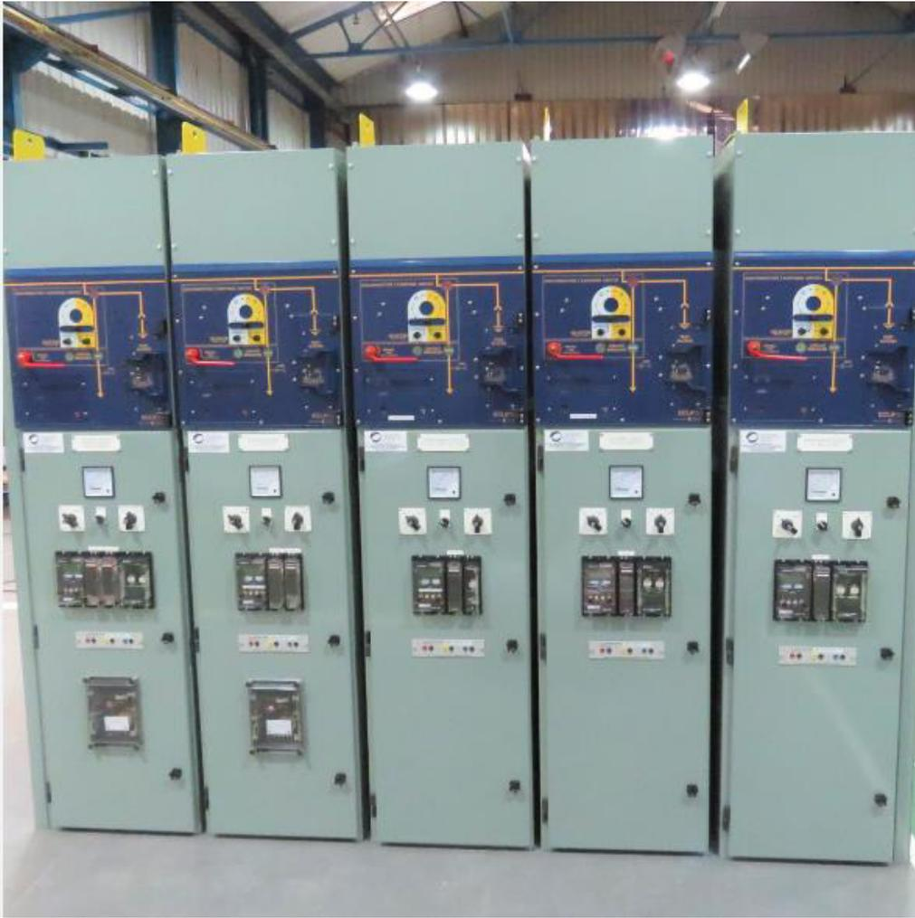
Figura 8 – HV switchgear
