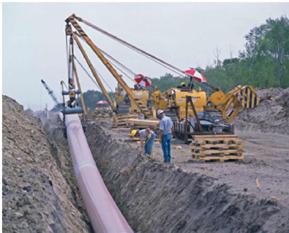
Fig. 9 – Posa in trincea
