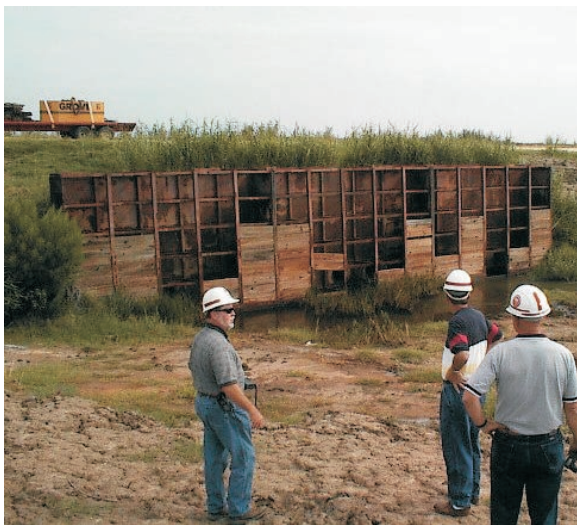
Figure 4. Weir boards in large weir, Blakeley Island site
