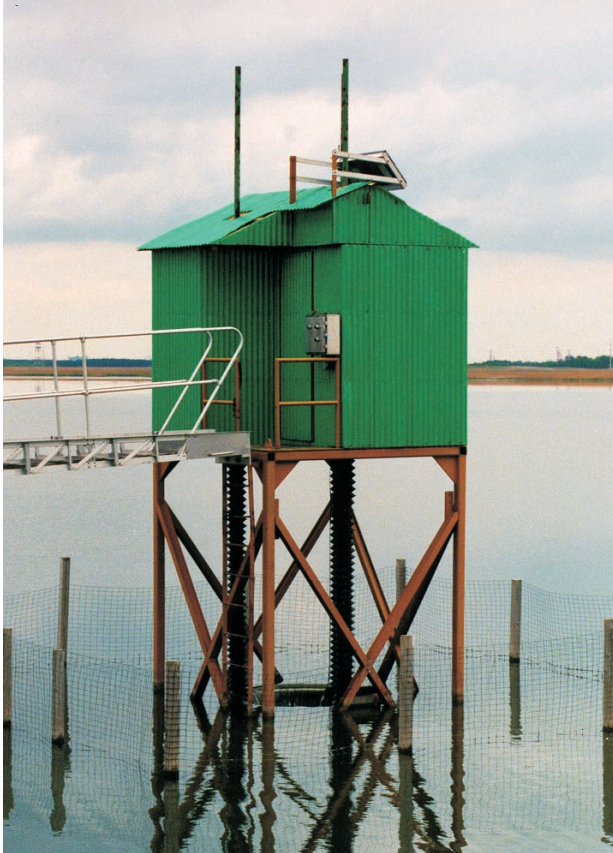
Figure 9. First weir installed at Craney Island CDF
