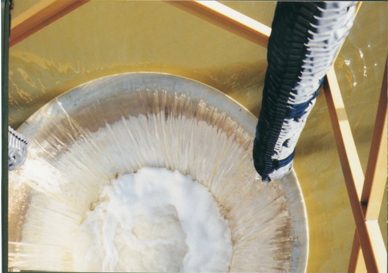
Figure 12. Clear waters flowing over telescoping weir crest
