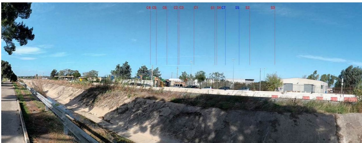
Vista 3_2 post operam
