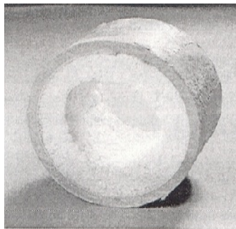
Figure 14. Clogged pipe from a tunnel site due to leaching of Ca(OH) 2 .
