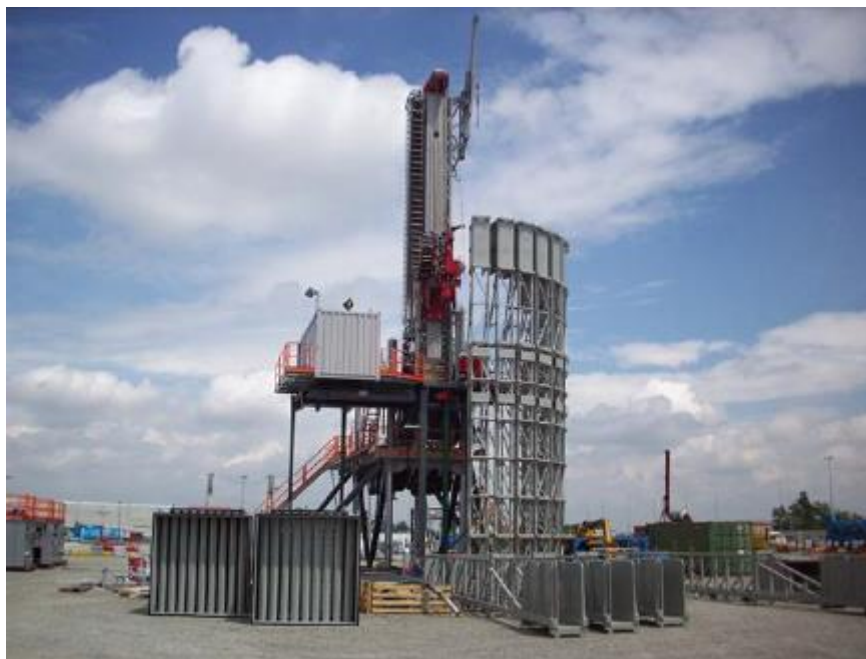
Figura 3-E: Impianto Drillmec HH-200MM
