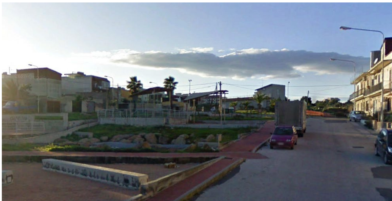
FOTO 12 ANTE OPERAM - VILLASMUNDO Via Cavour
