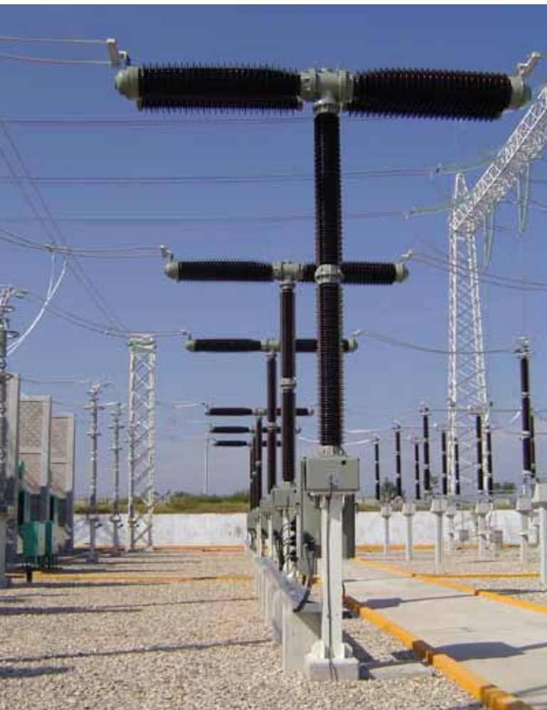
3AP2 FI 420 kV Live-tank circuit-breaker in operation at a major power transmission and distribution company
