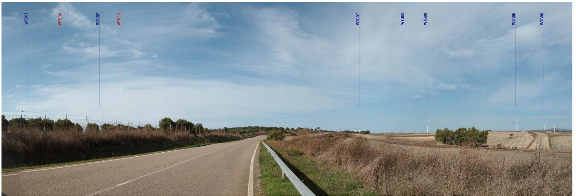
Vista 11_1 post operam
