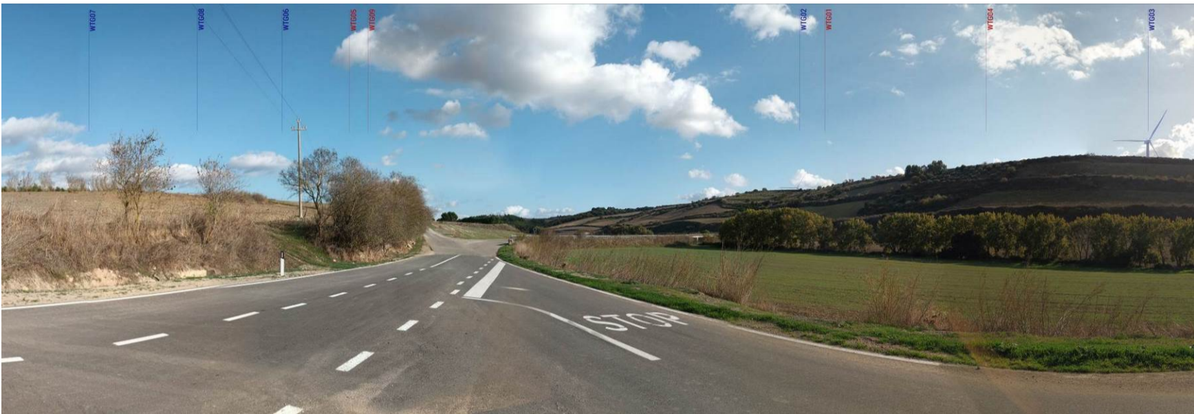
Vista 4_2 post operam
