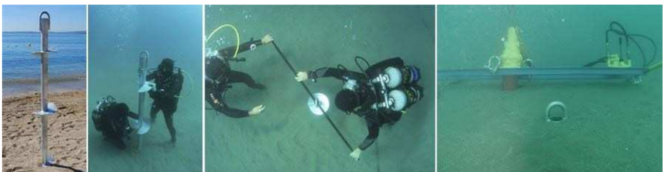
Figura 8. Screw anchor
