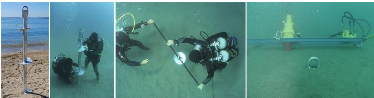
Figura 7. Screw anchor
