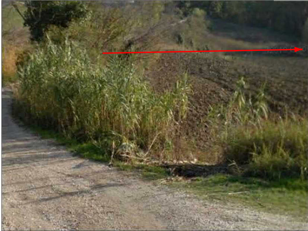
Area cantiere microtunnel "Castorano"
