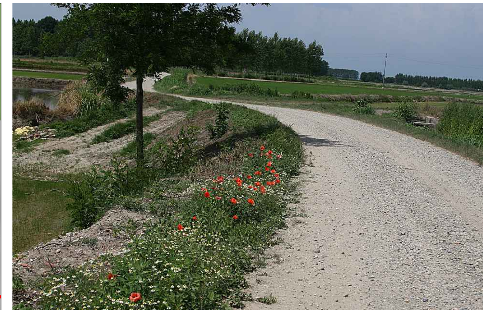
Strada in Macadam
