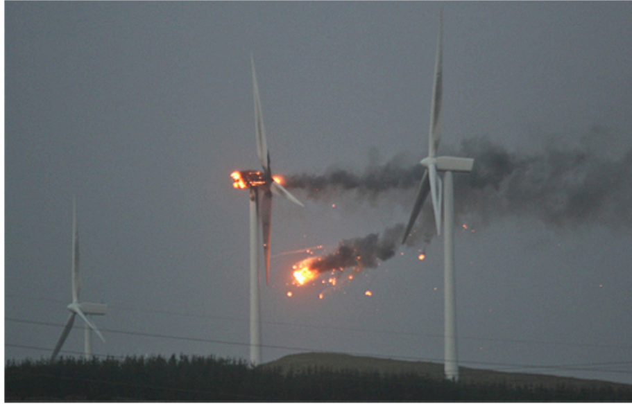
Fig. 5. Wind turbine fire at Ardrossan wind farm [17].
