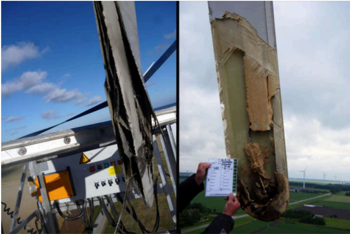
Figure 6. Images of wind turbine blade shell detachment.
