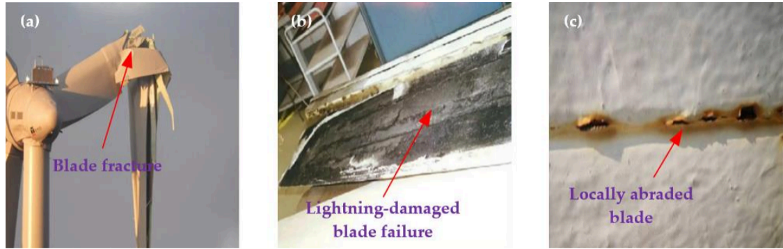
Figure 4. Forms of blade failure. (a) Blade fracture accident caused by design flaw [24]; (b) lightning-damaged blade failure [30]; (c) locally abraded blade [34].
