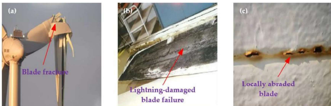
Figure 4. Forms of blade failure. (a) Blade fracture accident caused by design flaw [24]; (b) lightning-damaged blade failure [30]; (c) locally abraded blade [34].
