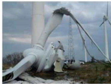
(a) Collapsed nacelle
