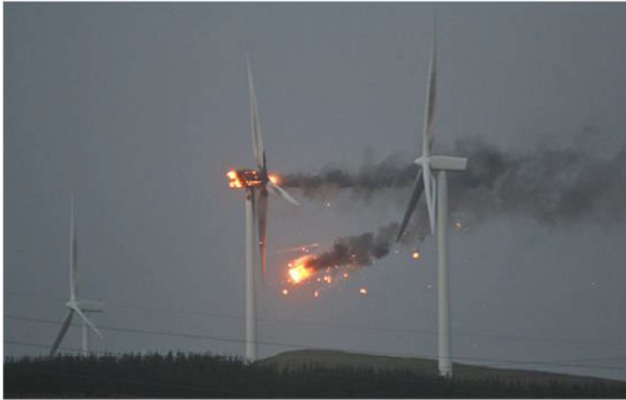
Fig. 5. Wind turbine fire at Ardrossan wind farm [17].
