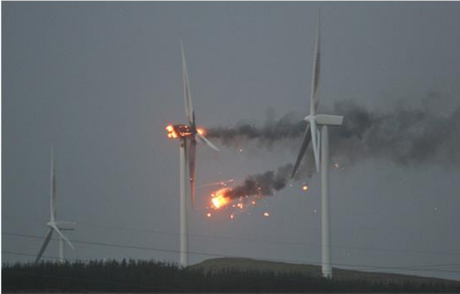
Fig. 5. Wind turbine fire at Ardrossan wind farm [17].
