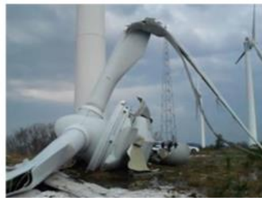
(a) Collapsed nacelle
