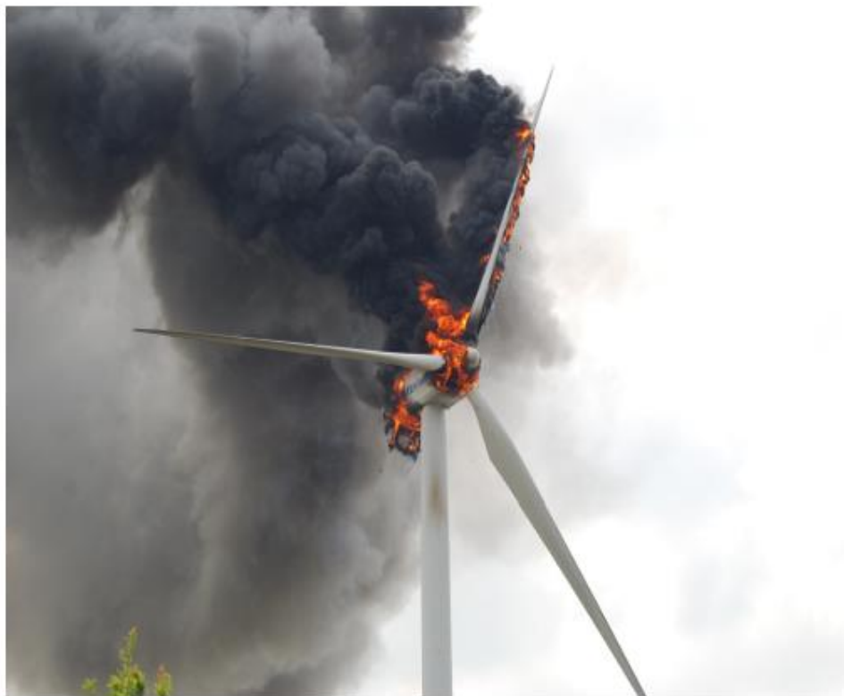
Fig. 6. Wind turbine on fire at the Groß Eilstorf wind farm [22].
