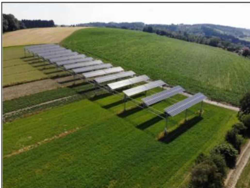
*Figura 43: Scientific APV power plant from above with reference area next to it and in operation in 2018, producing Demeter-certified organic potatoes, winter wheat, clover, and celery*
