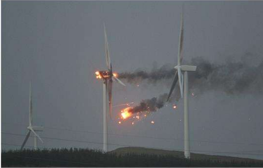
Fig. 5. Wind turbine fire at Ardrossan wind farm [17].
