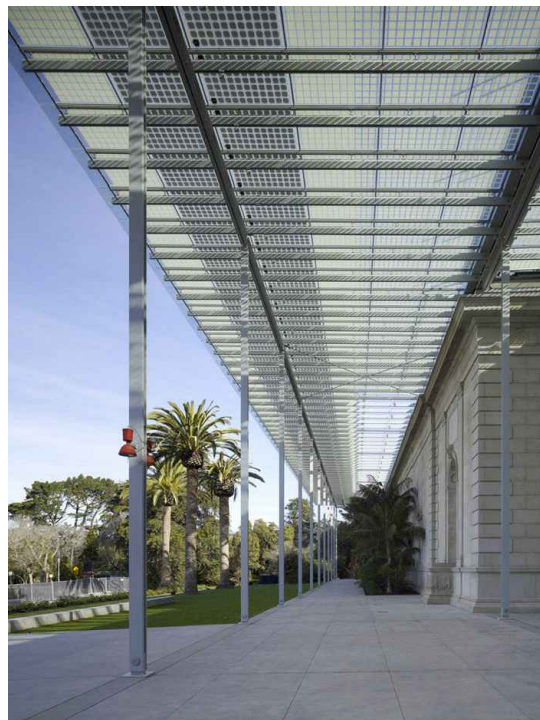
Renzo Piano Building Workshop, San Francisco
