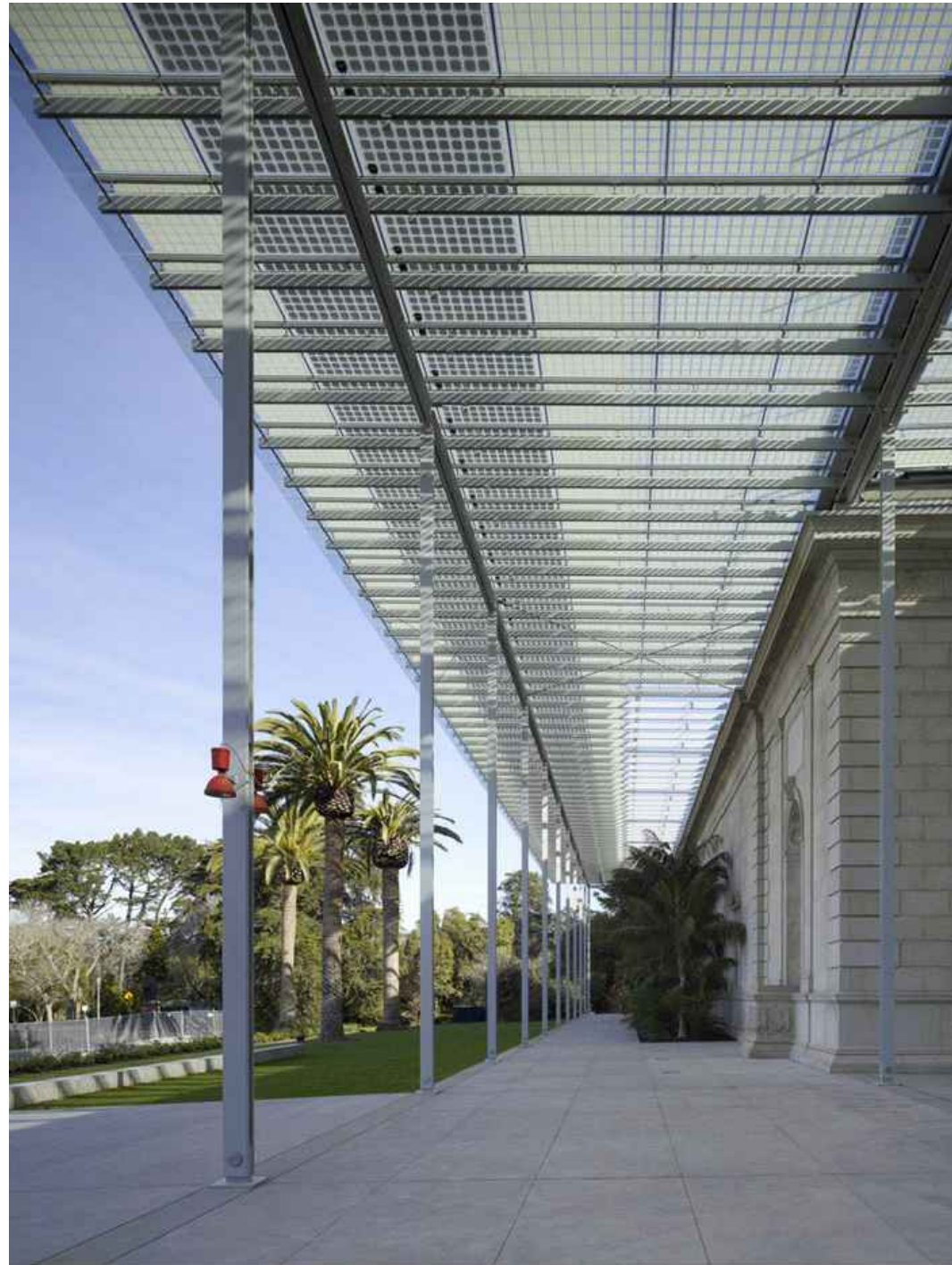
Renzo Piano Building Workshop, San Francisco
