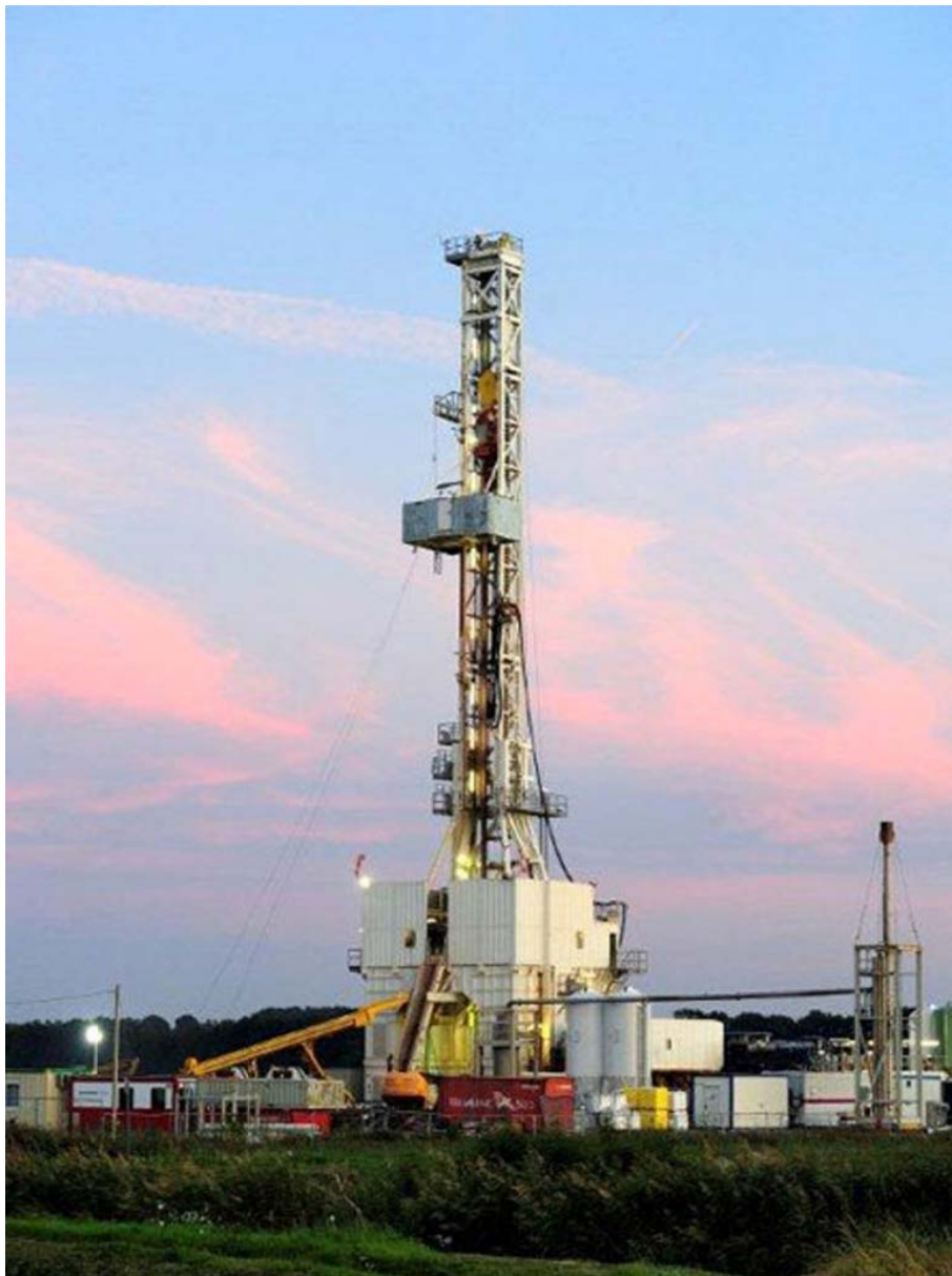
Figura 14. Impianto HH 220 DRILLMEC.
