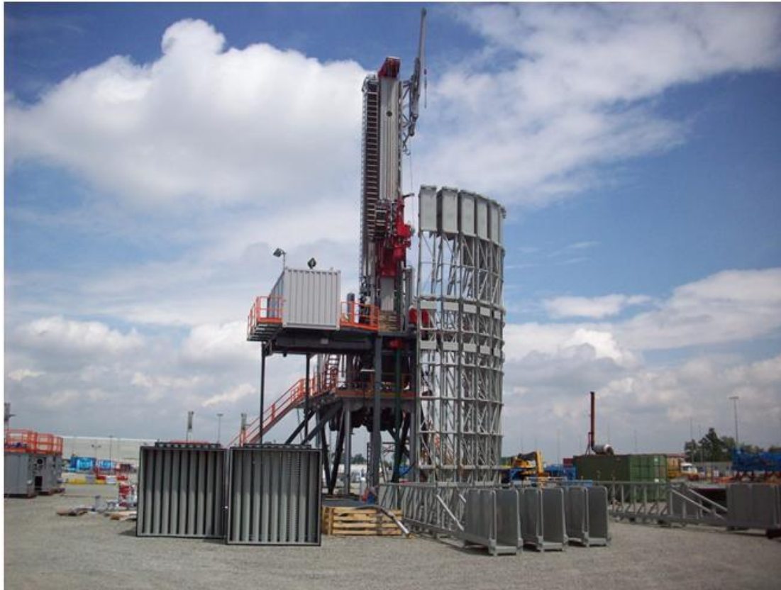
Figura 2 RIG DRILLMEC HH200MM (LP Drilling)
