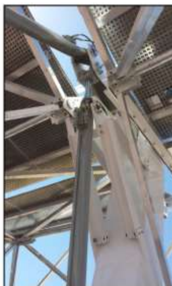
Figura 14. Drive & tracker Pylon LAT 8.0 m – Pistoni in serie
