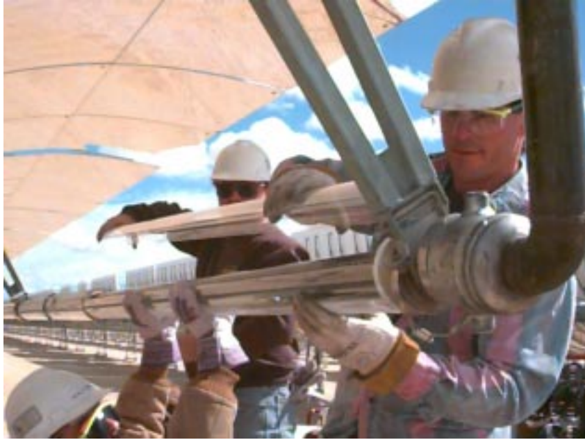
Figure 5. Split-glass envelopes were developed as a temporary method of reducing HCE heat losses.
