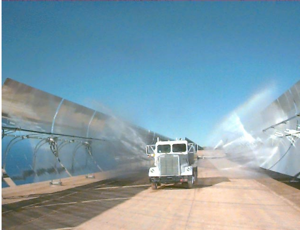
Figure 9. A truck can be used to apply a “deluge-type” stream of water to parallel rows of mirrors.
