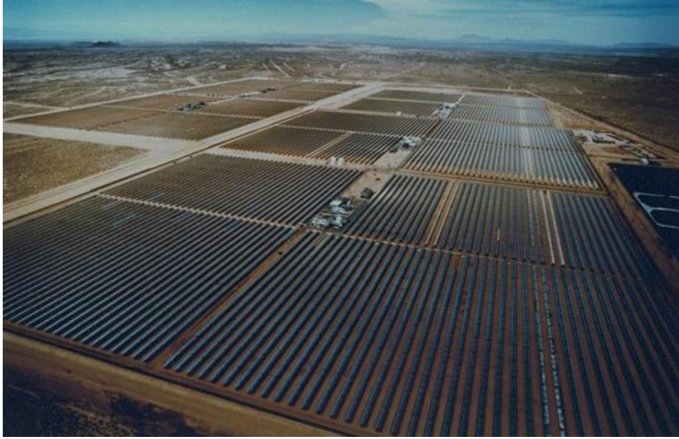
Figure 1. The Kramer Junction power park is comprised of five 30-MW plants.
