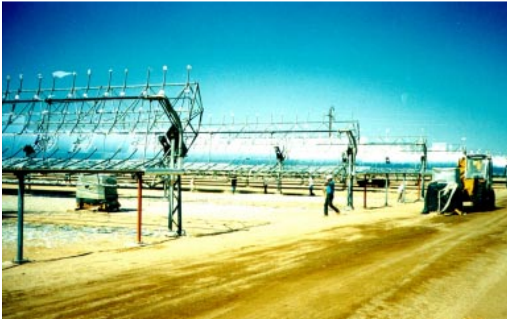
Figure 10. Mirror damage typically occurs along the edge of a solar field. In the worst-case event shown above, a tornado hit Kramer Junction on July 29, 1995.
