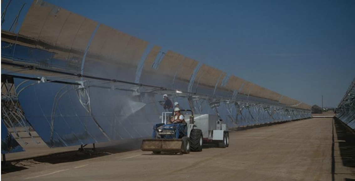
Figure 7. In the traditional method, high-pressure demineralized water is sprayed on the mirrors with hand-held nozzles.
