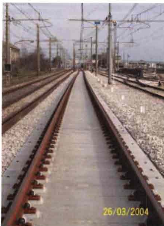
Figura 42 - MAX BÖGL – HIPERTRACK – SLAB - TRACK SYSTEM ( h = 200 mm )
