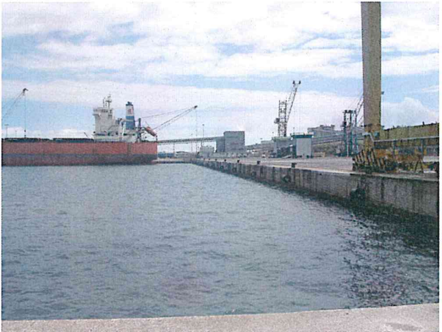
Panoramica banchina Costa Morena
