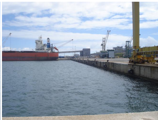
Panoramica banchina Costa Morena
