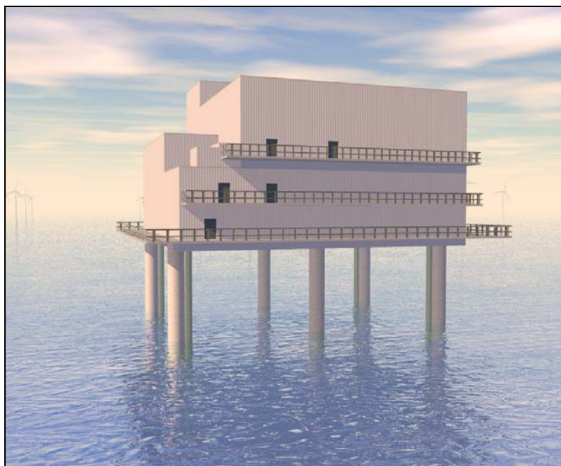
Figura 2-12 Electric Service Platform offshore
