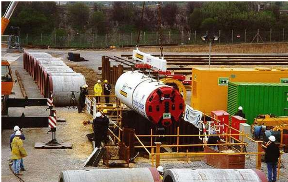
Fig. 8.2 – Microtunnel construction yard
