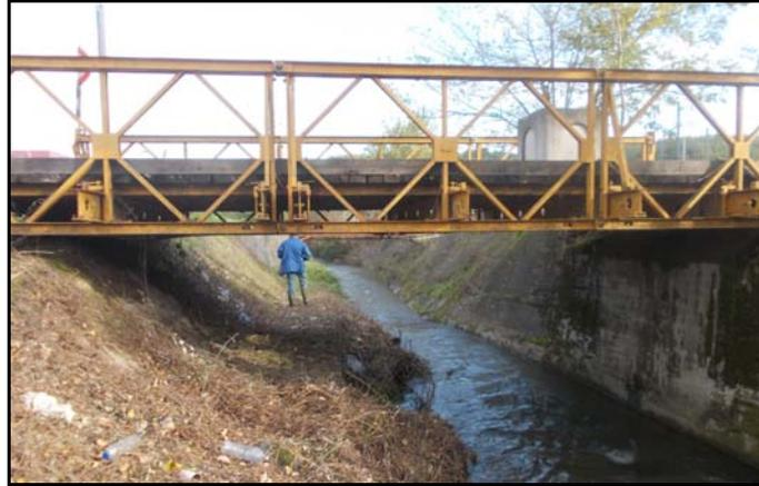
FIGURA 19 - PONTE METALLICO TIPO BAILEY
