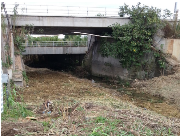
ANTE OPERAM – area intervento 3
