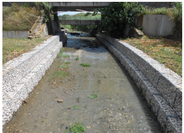
POST OPERAM – area intervento 3
