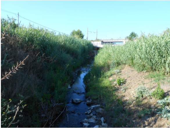
ANTE OPERAM – area intervento 1
