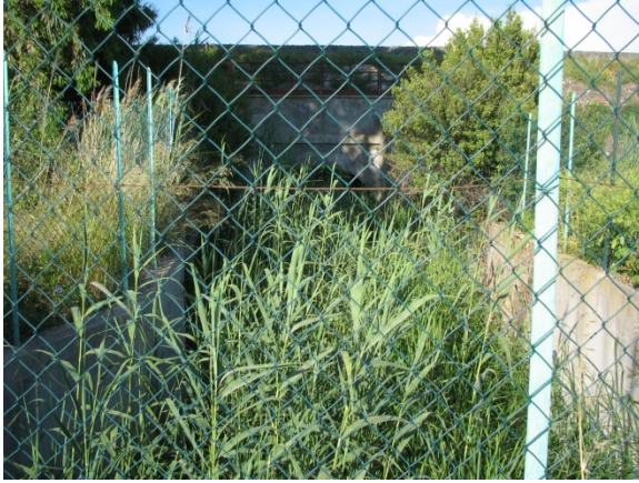
ANTE OPERAM – area intervento 6
