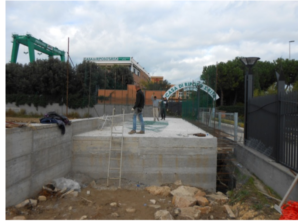
POST OPERAM – area intervento 6
