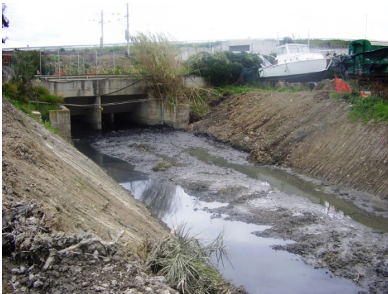
ANTE OPERAM – area intervento 8
