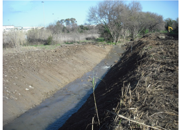
POST OPERAM – area intervento 1
