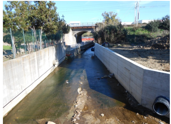
POST OPERAM – area intervento 13
