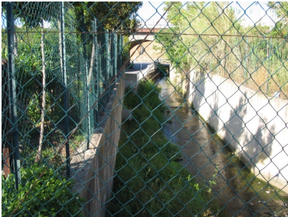
ANTE OPERAM – area intervento 13
