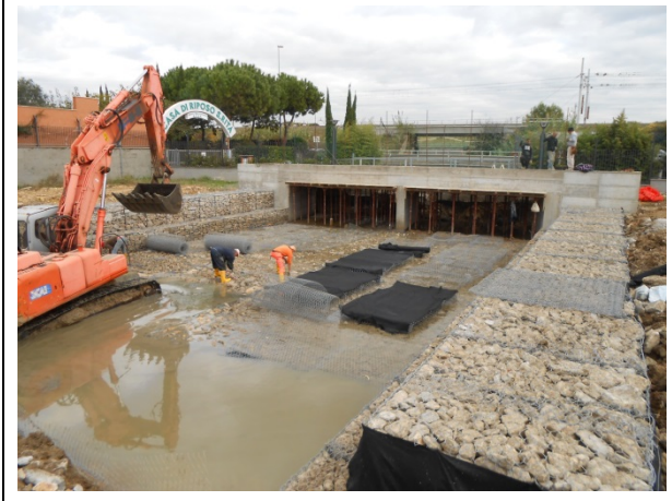
POST OPERAM – area intervento 7
