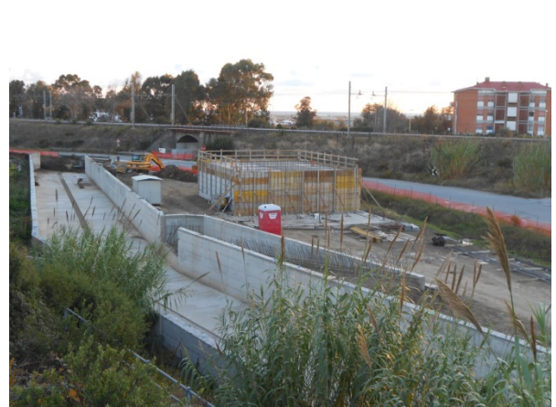
POST OPERAM – area intervento 9
