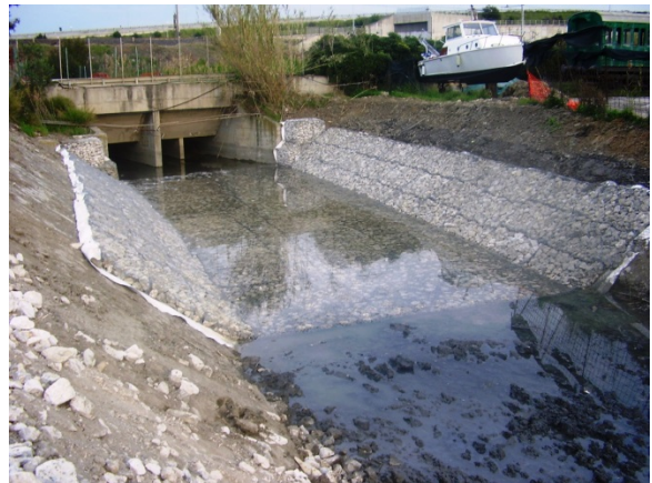
POST OPERAM – area intervento 8
