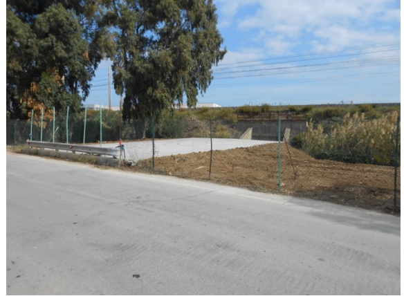
POST OPERAM – area intervento 6
