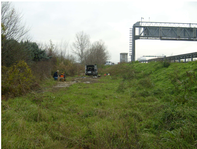
Area cantiere cross hole
