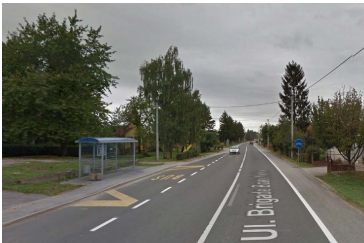
Figure 44: A well-equipped bus stop outside the agglomeration (Source GoogleMaps)
