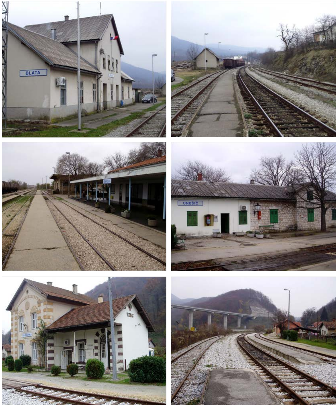
Figure 51: Examples of the security problems at the stations in rural areas Blata, Benkovac, Unešić and Durmanec (no surveillance systems, lights, unsecure access paths)
