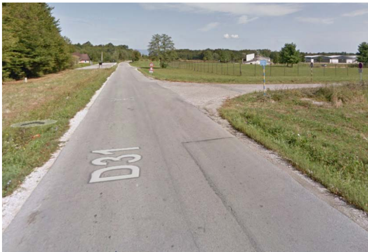
Figure 43: A typical bus stop on Croatian roads outside the agglomeration (Source GoogleMaps)
