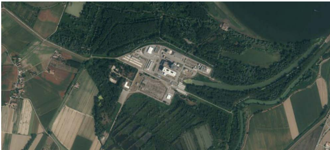
Figure 2.1-2: Caorso nuclear power plant
