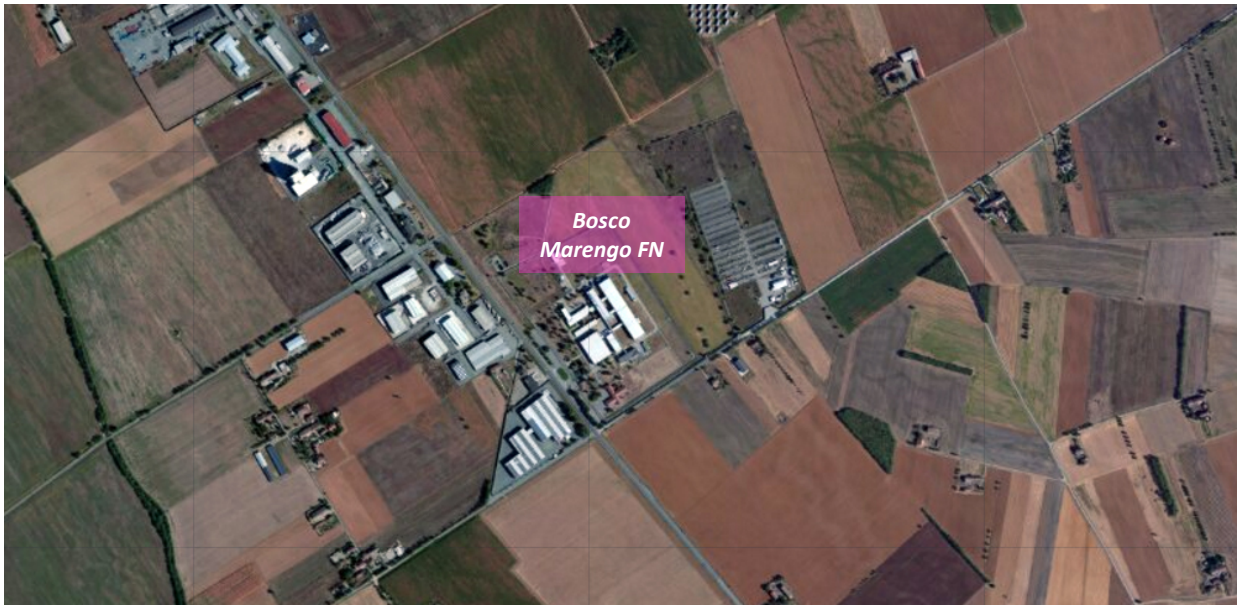
Figure 2.1-5: Bosco Marengo FN plant
