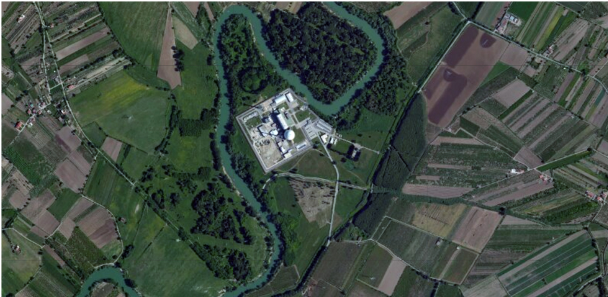
Figure 2.1-4: Garigliano nuclear power plant
