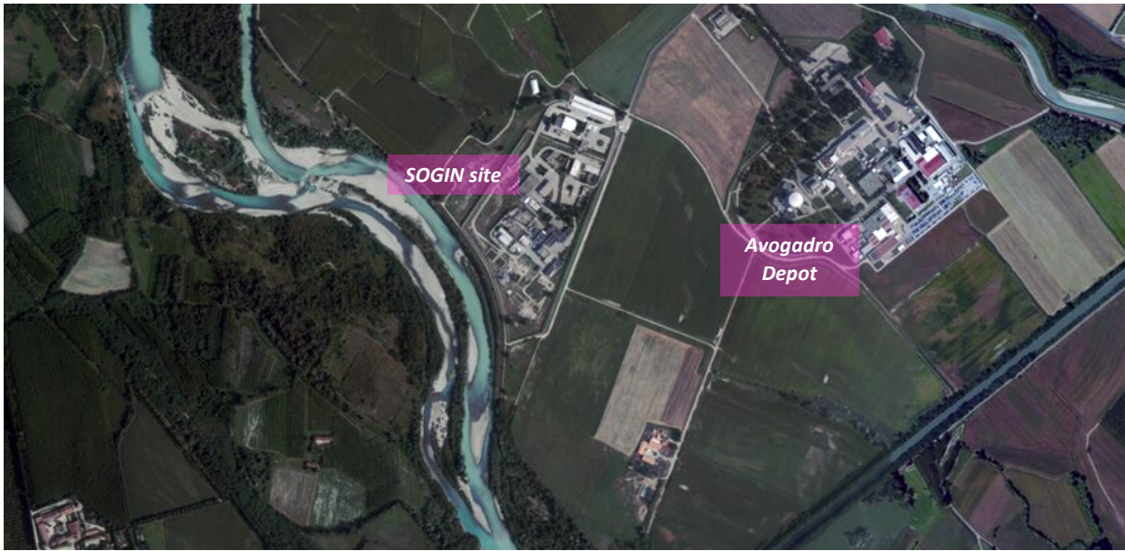
Figure 2.1-6: Saluggia nuclear complex
