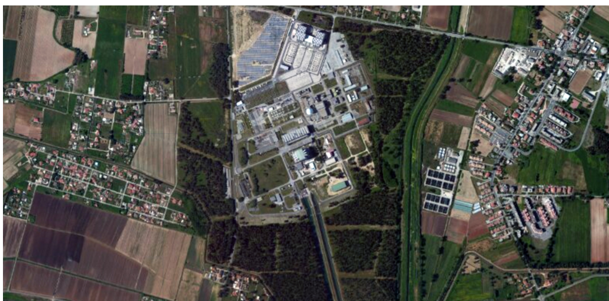
Figure 2.1-3: Latina nuclear power plant
