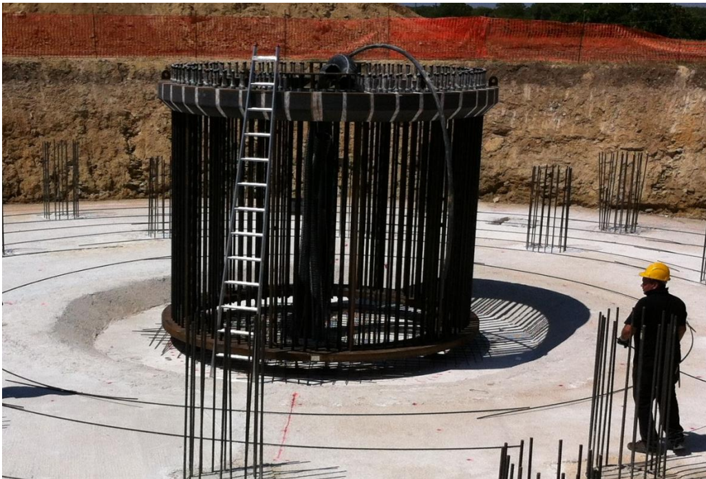
Fig. 2.7 - Anchor Cage
