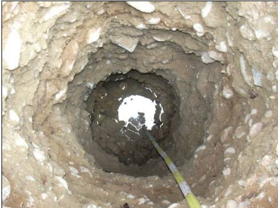
Figura.17 Prescavo MW05 (2,1m)
