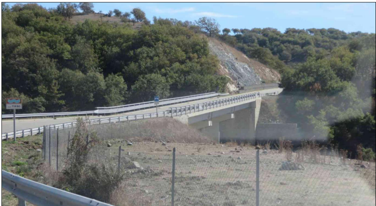
Observation n. 20: Bridge on SP 107
