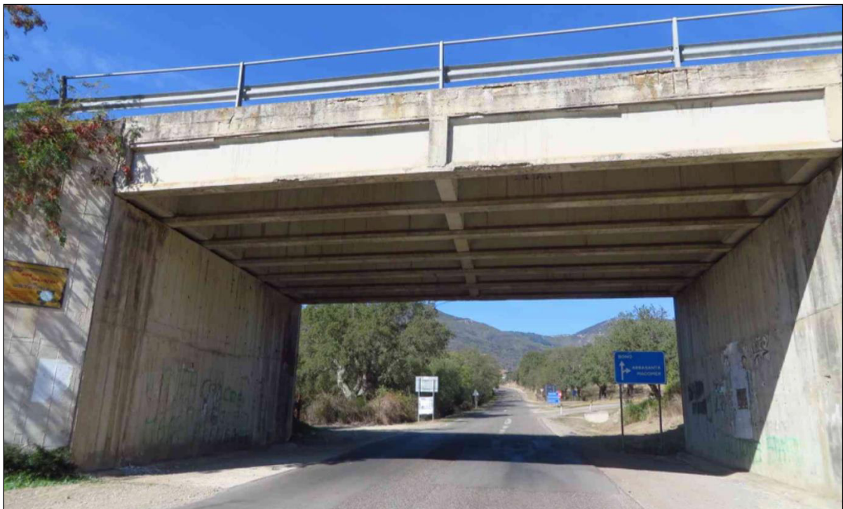
Observation n. 12: Bridge on SP 33
