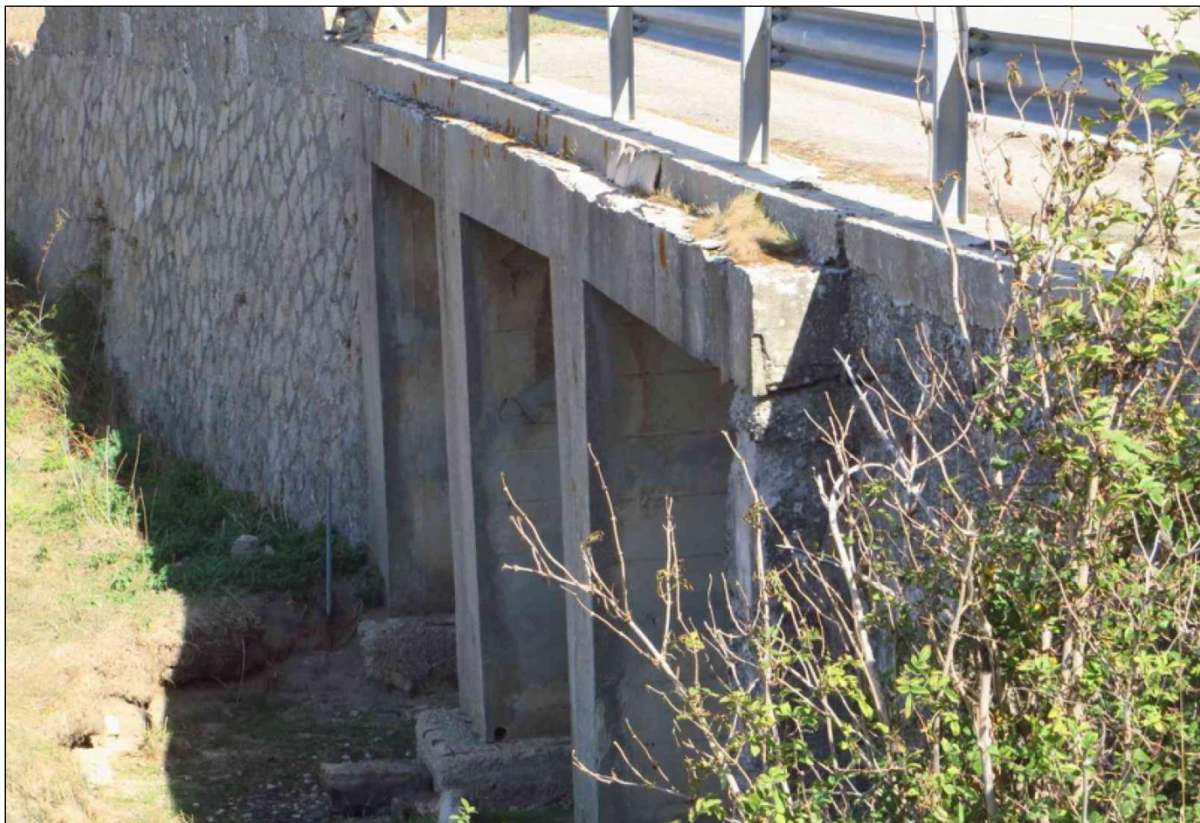
Observation n. 19: Bridge on SP 32
