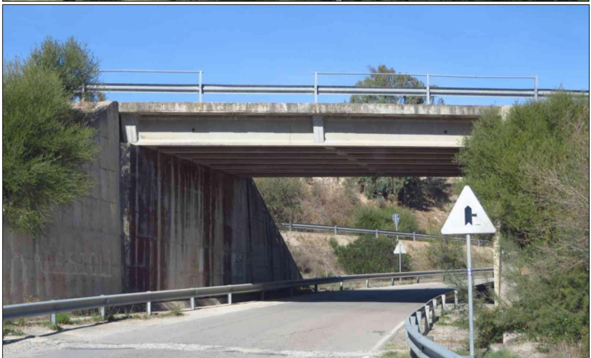
Observation n. 18: Bridge on SP 33
