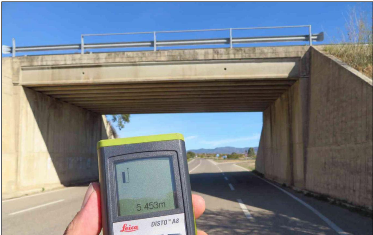
Observation n. 13: Overbridge on SP 33
