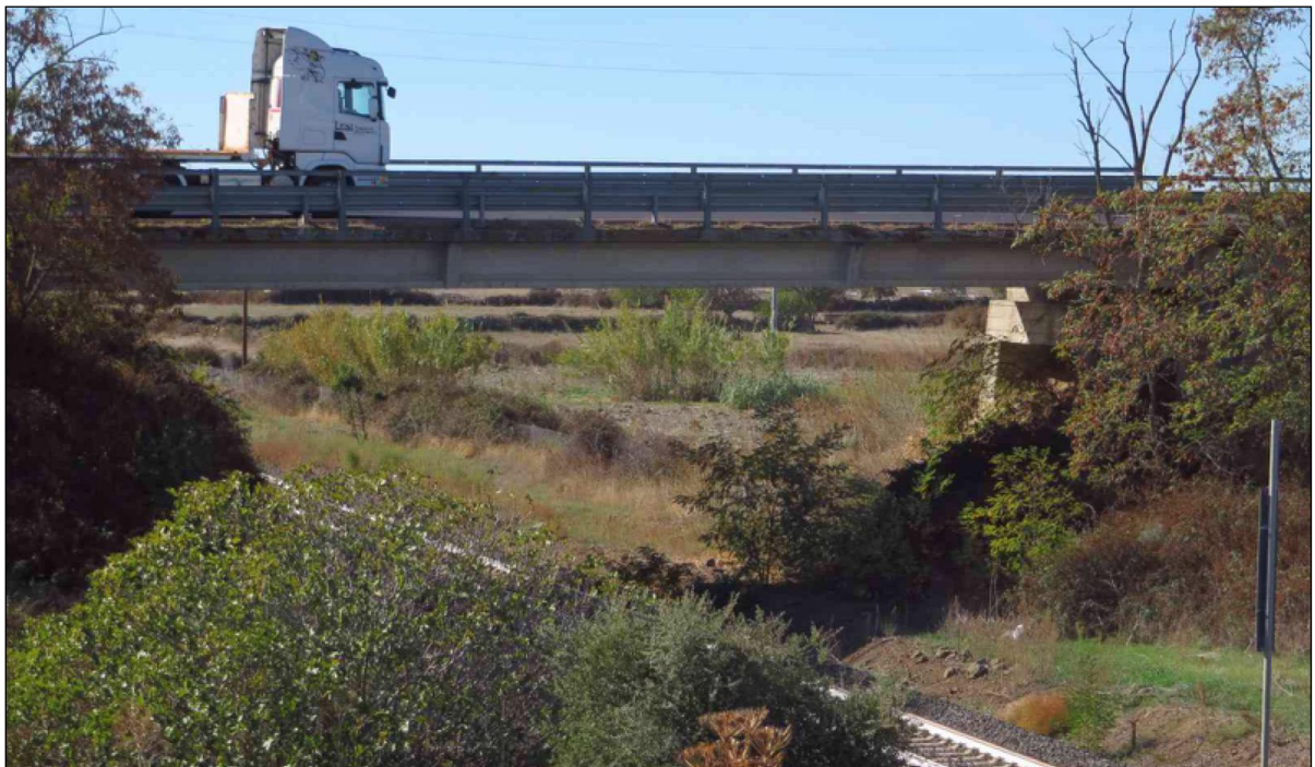
Observation n. 1: Bridge on SP 33
