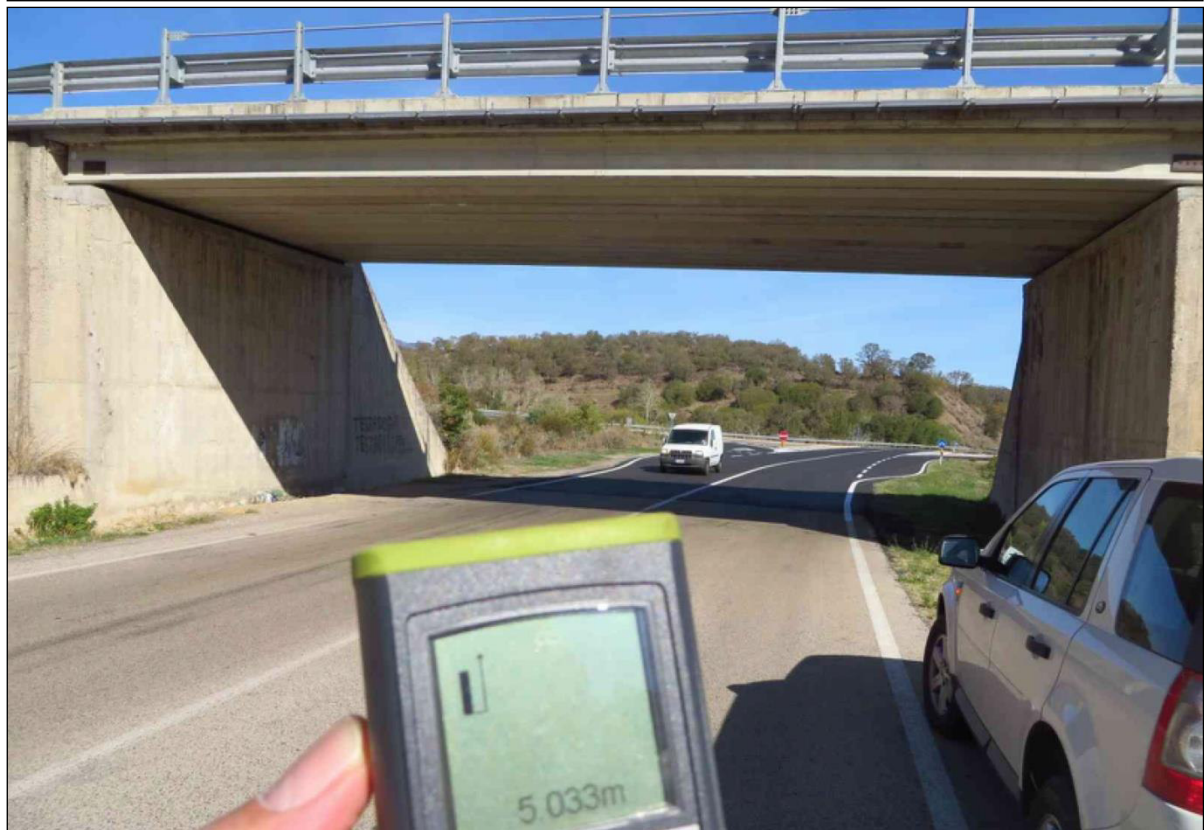
Observation n. 10: Overbridge on SP 33
