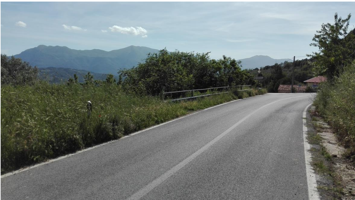
Strade – Conglomerato bituminoso
