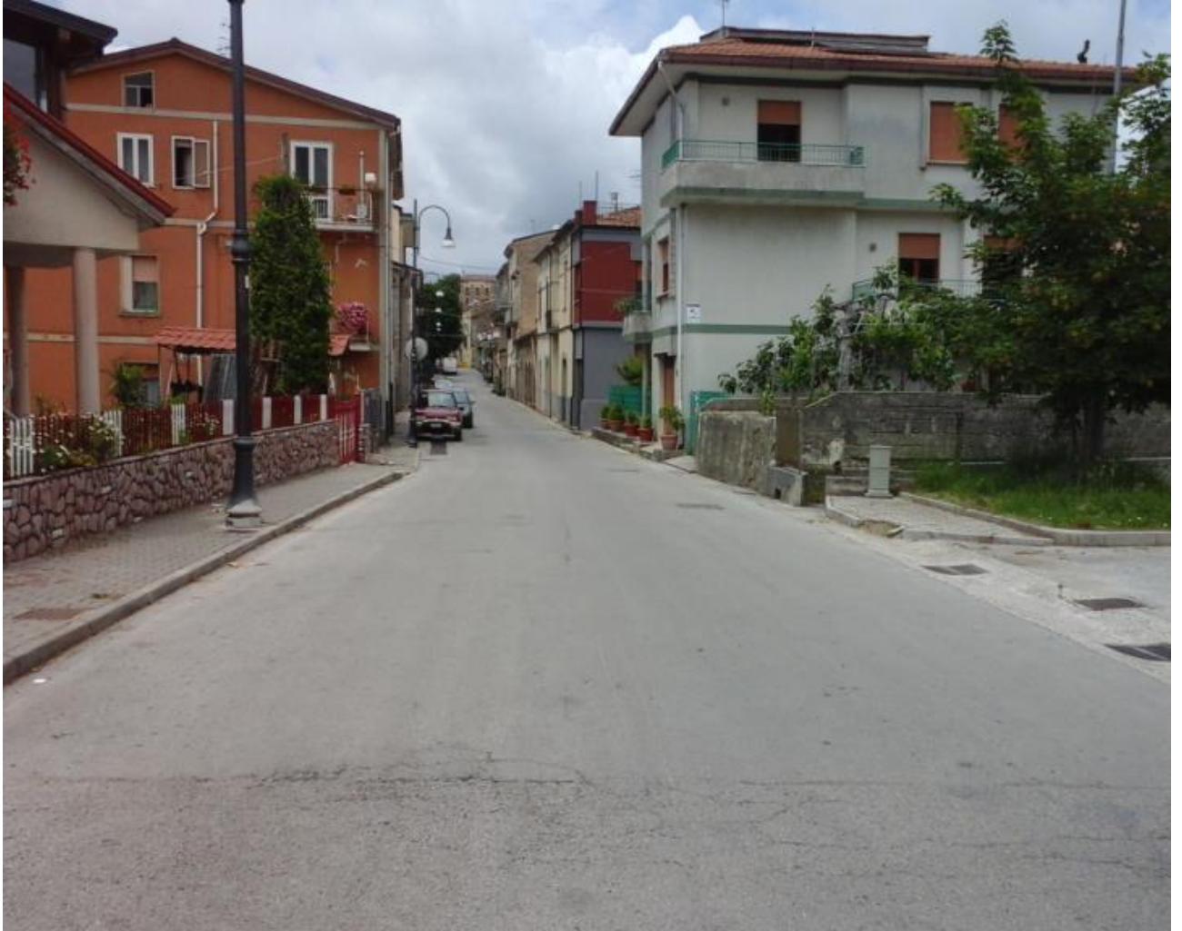
Strade – Conglomerato bituminoso
