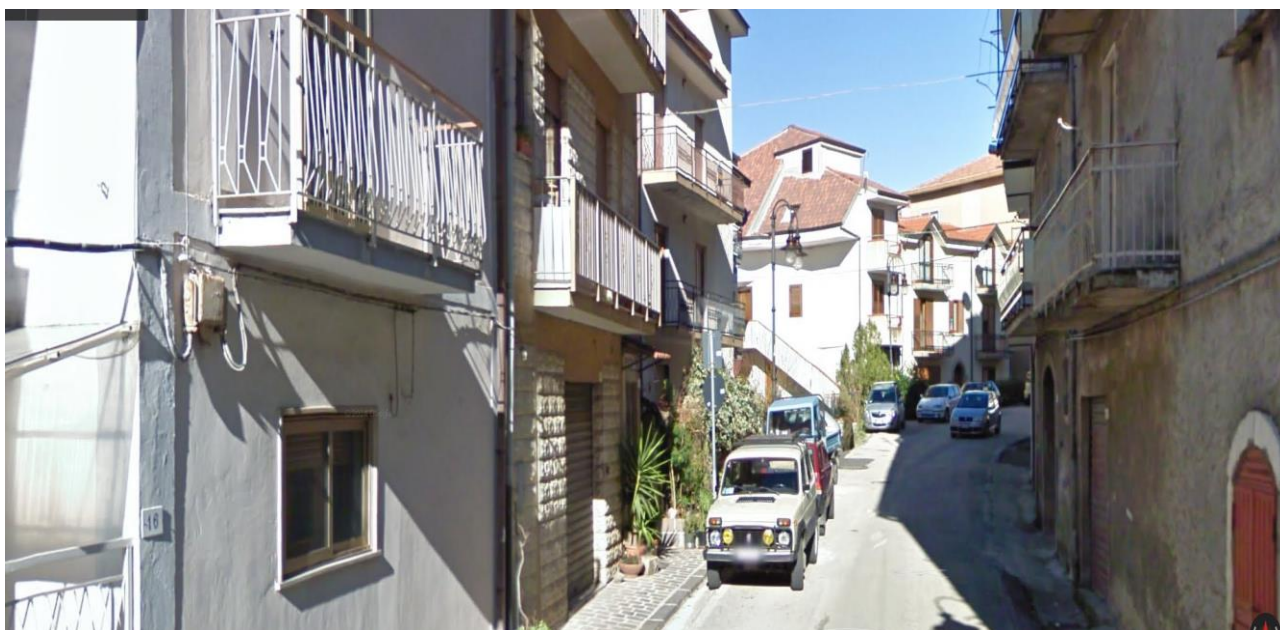
Strade – Conglomerato bituminoso
