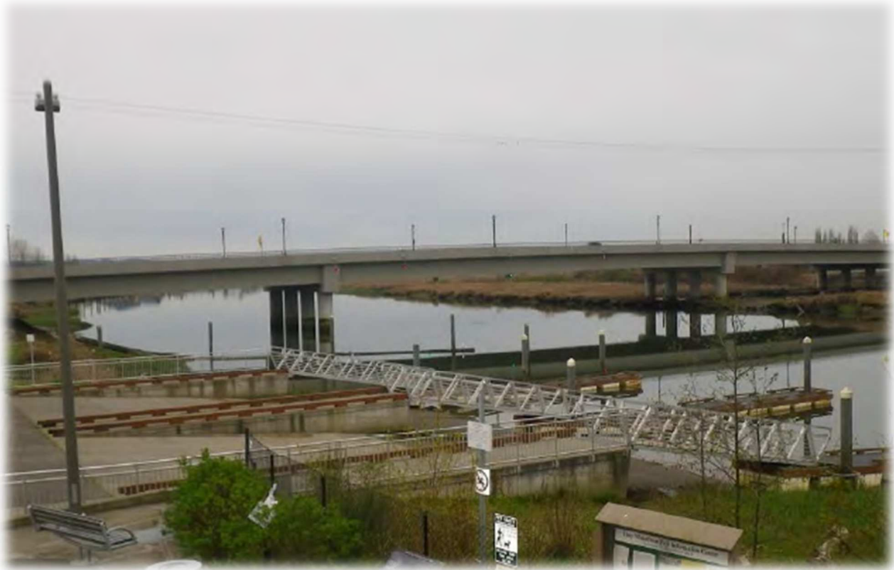
Figura 12 – Ebey Slough Bridge
