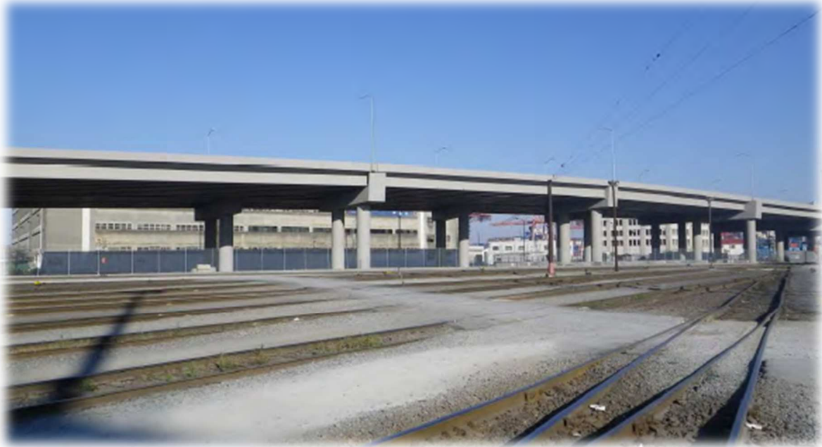
Figura 10 – Alaskan Way Viaduct
