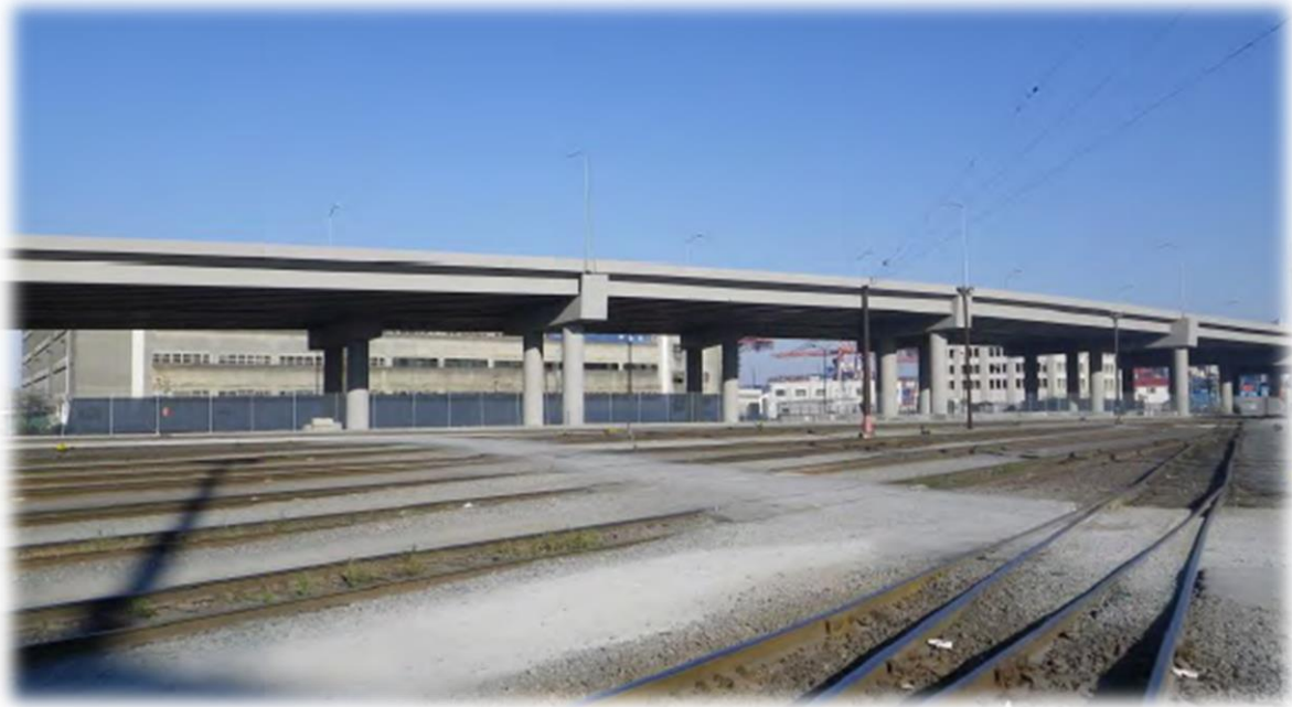
Figura 12 – Alaskan Way Viaduct
