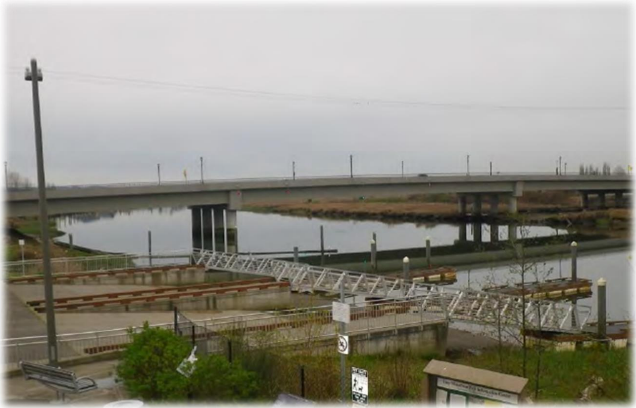
Figura 14 – Ebey Slough Bridge
