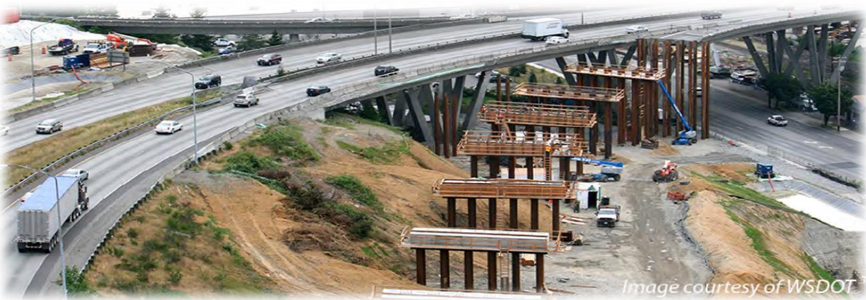
Figura 15 – Eastbound Nalley Valley Bridge
