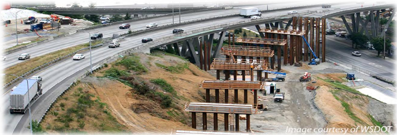
Figura 14 – Eastbound Nalley Valley Bridge
