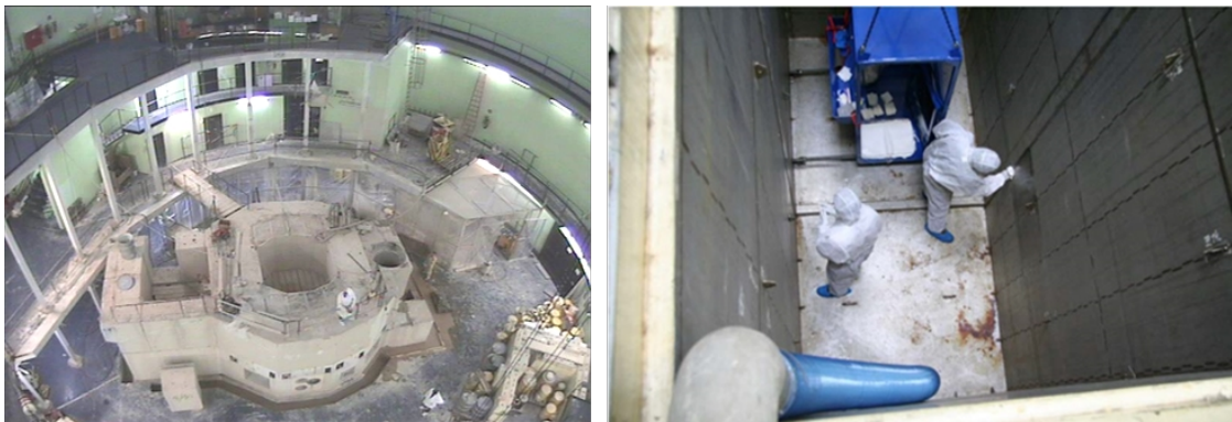
Figure 2: Dismantling the research reactor ASTRA and the spent fuel pool
