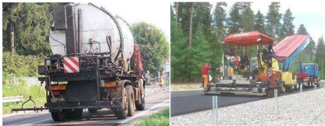
FIGURA 5-2 – A SX APPLICAZIONE DI EMULSIONE BITUMINOSA, A DX VIBROFINITRICE
