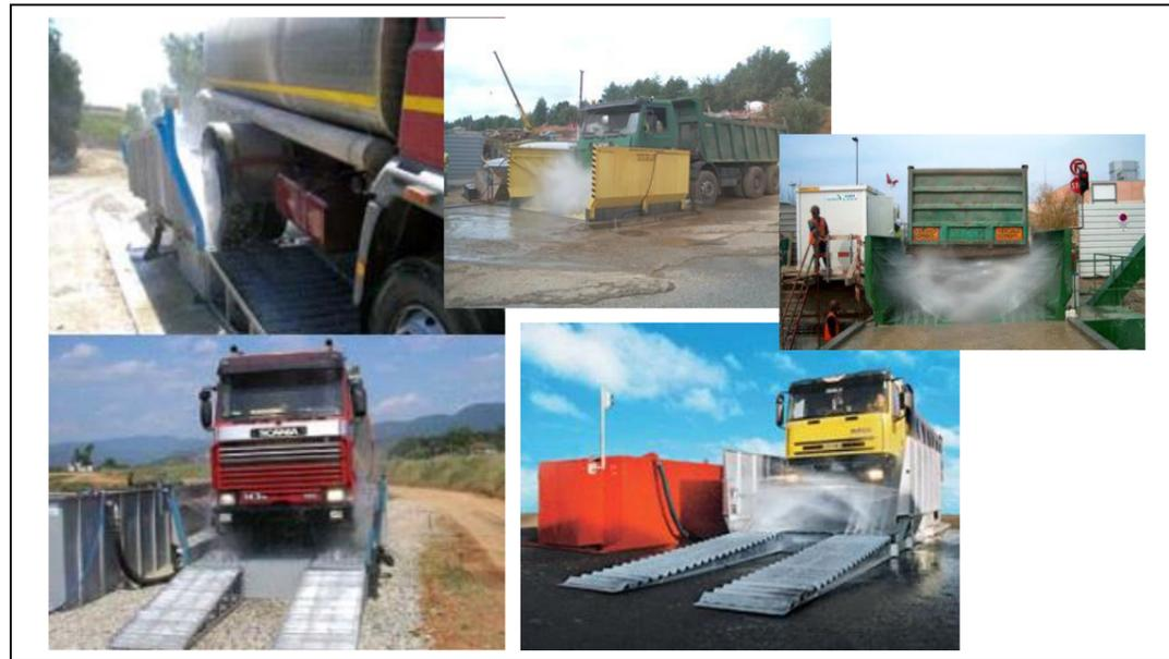
FIGURA 6-9 – SISTEMI PER IL LAVAGGIO DEI PNEUMATICI AD ALTA PRESSIONE
