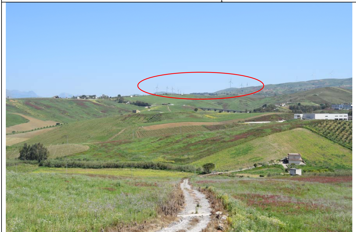
Foto 2 – EXSS113 – post operam
