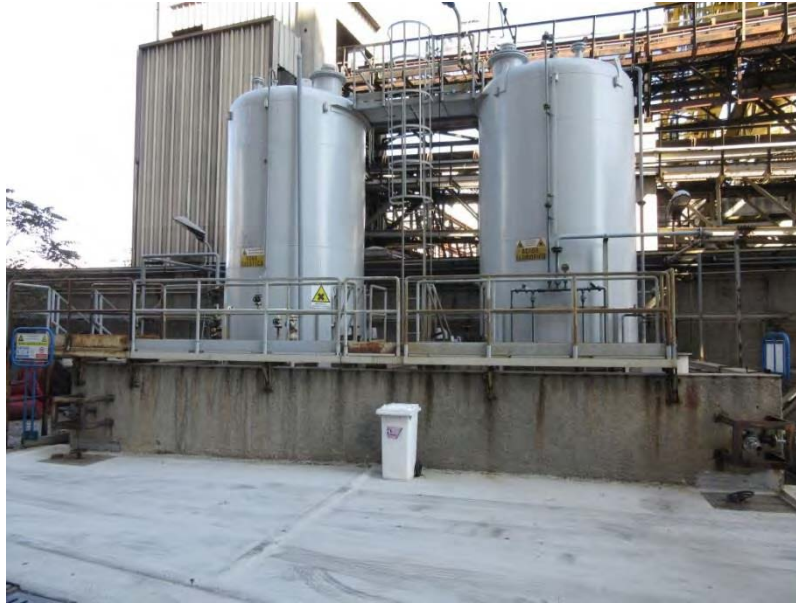
Figura 13: serbatoi HCl e NaOH
