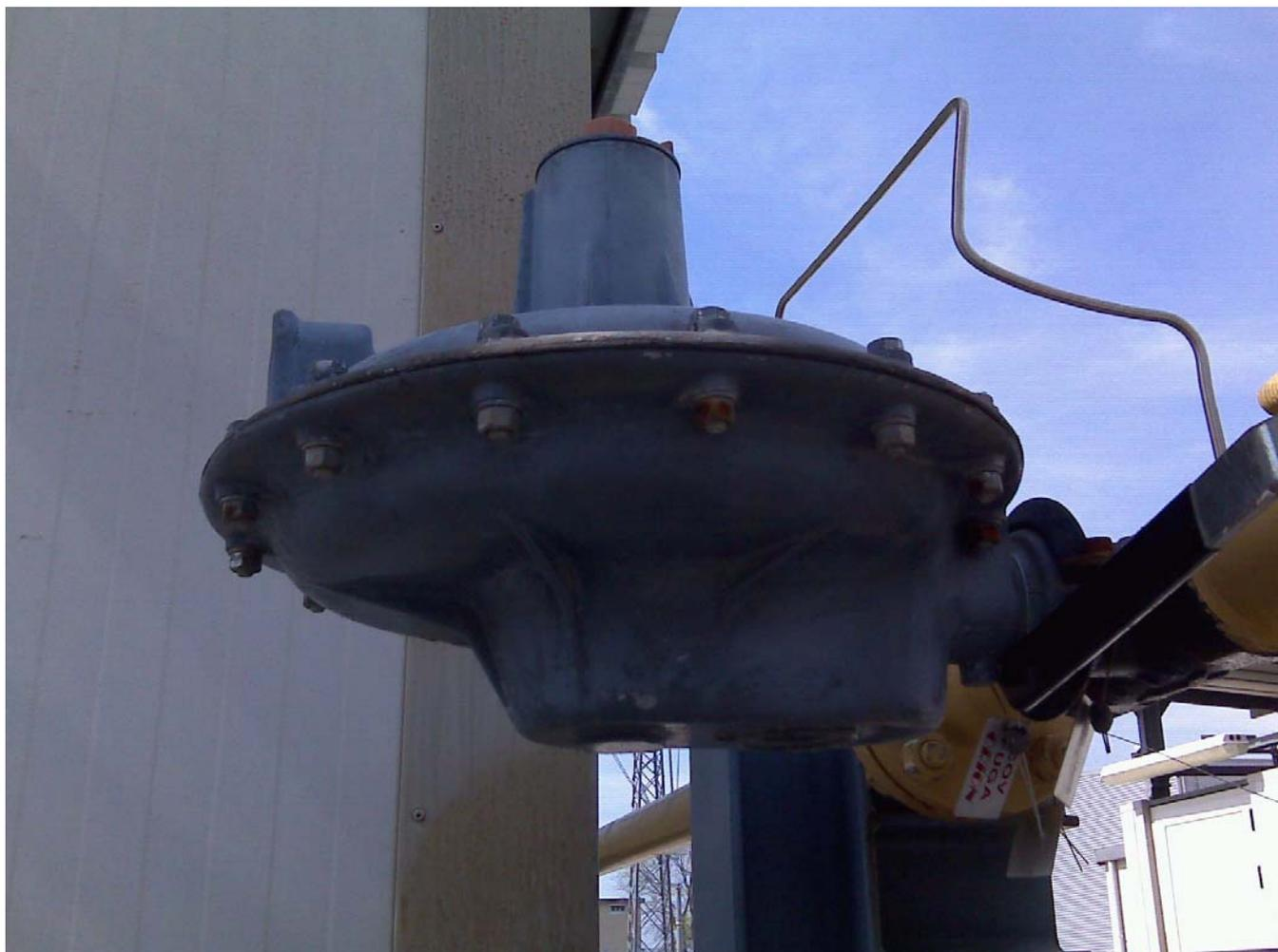
4) DALLA VALVOLA 10EKD14AA053 , INVIO FUEL GAS A WATER BOILER E HVAC
