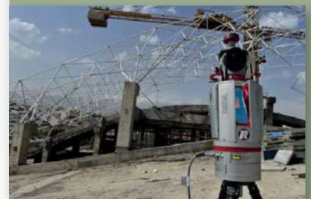
construction site monitoring
